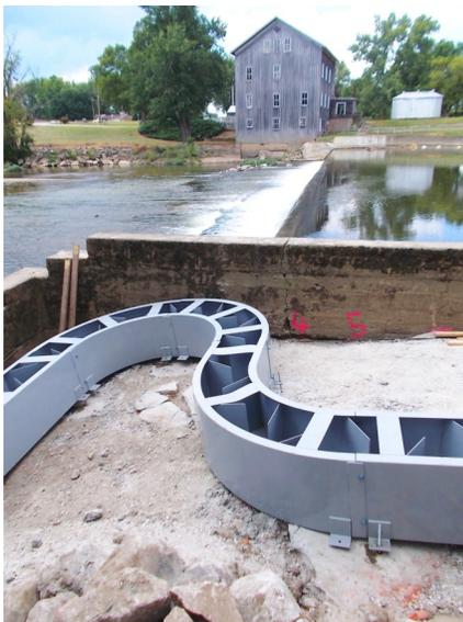
“tube” was assembled. Headwall and foot-wall extensions, with openings for the ladder, were added to the existing wall. The entire ladder was then encased in concrete. Site engineer Martin Duffy then relocated ballast boulders, that had long ago been placed behind the wall, for new uses in landscaping and water flow control.
