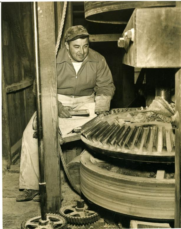
Addison Krom is shown repairing wooden cogs on a turbine shaft in 1953.
